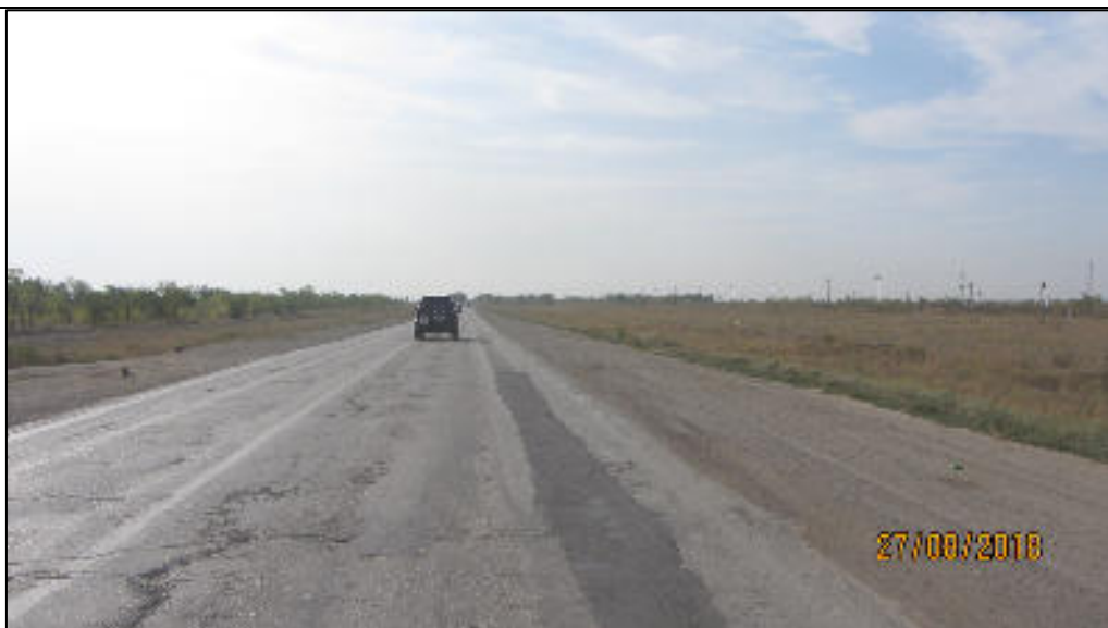
Plate B.2: KM13: Trees managed by the government adjacent to the road, but outside of the RoW.
