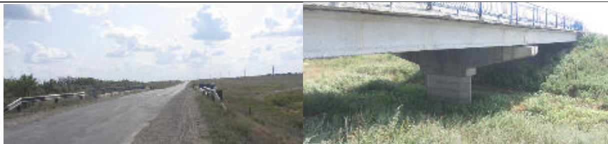
Plate B.23: KM52. Bridge – the riverbed is dry
