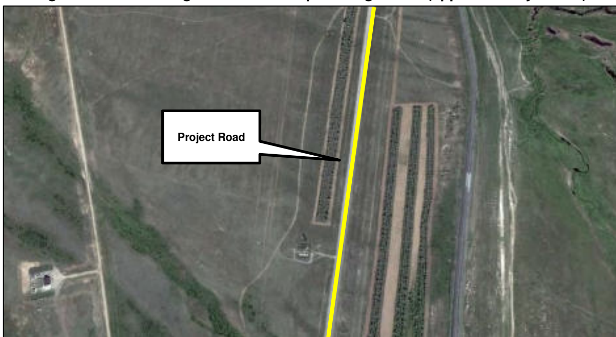
Figure 17: Aerial Image of Planted Strips of Vegetation (approximately KM 54)
