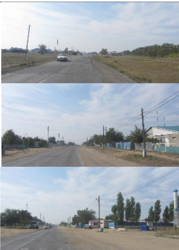
Plate B.9: KM 26+391–km29+40 : The most difficult part of the route passes within the boundaries of the Bestamak village. It is characterized by its passage in close proximity to residential houses, a large number of communications and networks, and junctions of secondary roads and spontaneous ramps 19 .
