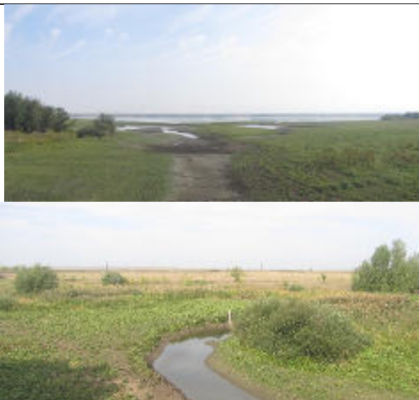
Plate B.4: KM18+561 – a three-span reinforced concrete bridge across the riverbed of the Kumsai River, flowing into the Aktyubinsk reservoir. The bridge, oriented from the north-west to the south-east, has a rectangular shape with dimensions of 54.6 × 8.15 m (length and width). The width of the roadway is 11.7 m, the height is 4.0 m. The roadway of the bridge is asphalt concrete, on both sides there are pedestrian walkways, protected from the roadway by concrete slabs with a height of 0.4 m. The edges of the bridge are 1.2 m.
