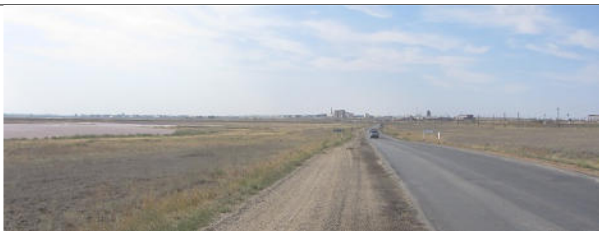
Plate B.17: KM40 + 84 -KM42 + 300 : there are wastewater (filtration fields) of the closed Alga chemical plant (the nearest distance from the road is 50 m, left side. The area of filtration fields currently is partially dry and covered by crust and vegetation, partially with water
